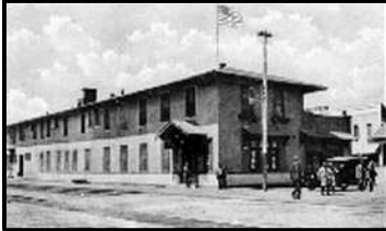
Harvey House, "Santa Fe Eating House".
